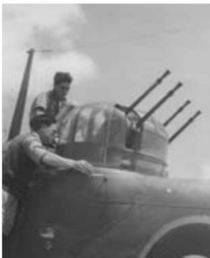
The Turret guns (four 0.303in) of a Mk III Baltimore. Here, LAC Gubbins (standing) and LAC Skill give them a check before flight.
